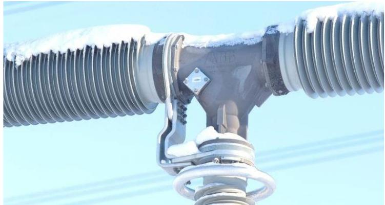
Fig. 8.5 TI montado en Interruptor (Figura Extraída de Smart Grids. FOCS solution with Digital Substation - ABB)
